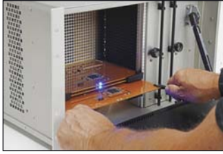
Installing an output expansion switch blade
